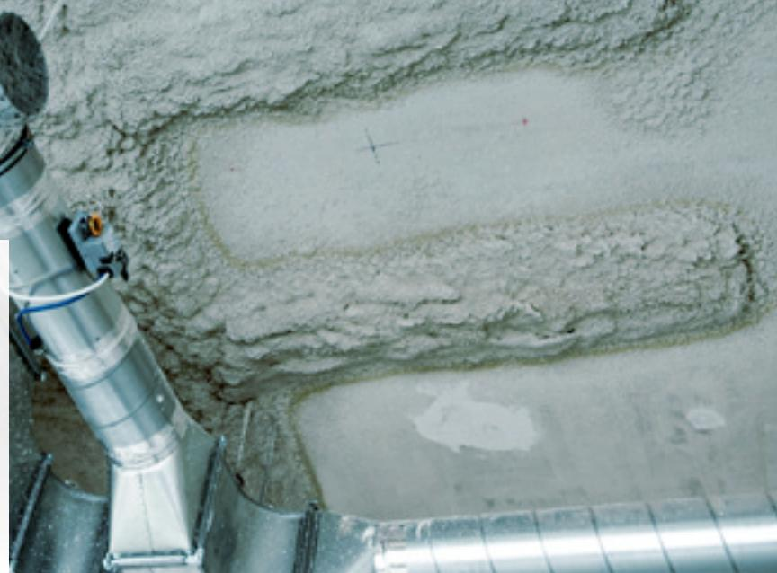
Knauf FP Vermiplaster has been developed specially for fire protection of buildings in interiors. Its task is to protect the load bearing coated construction elements in the event of a fire so that their function is maintained until the fire has been extinguished or building evacuated.
